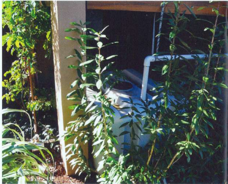
The Hurlbert's 250-gallon tank is filled to capacity after recent rains. The water, which used to run directly to the storm drain, is captured for slow release into this Indio Drive Ocean Friendly Garden.
